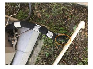
The receptacle has been tightened, however the cover plate cracked during the process... Owners advised they will replace plate.
