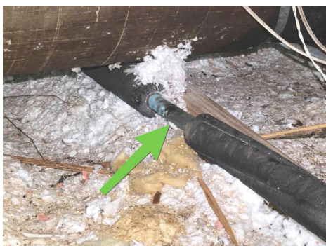
Condensation Leak
