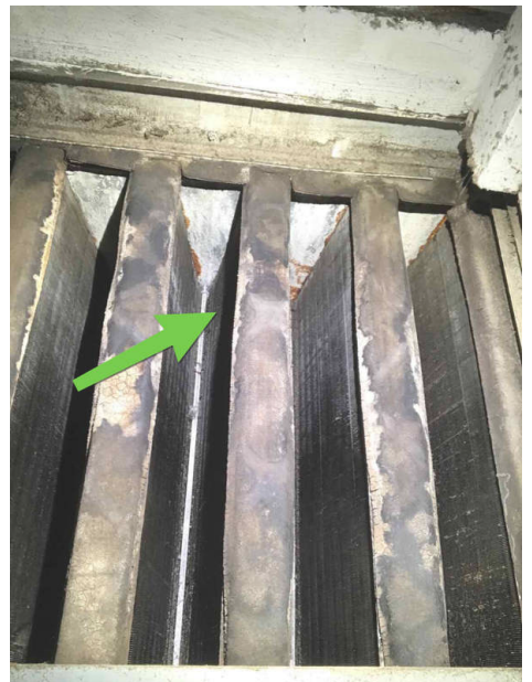
Mold Growth AC Coils
