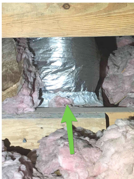
Cold Air Leak
