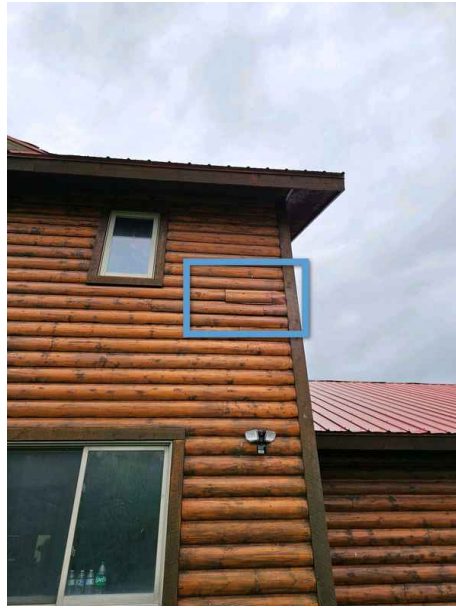
Repaired as of 5/29
