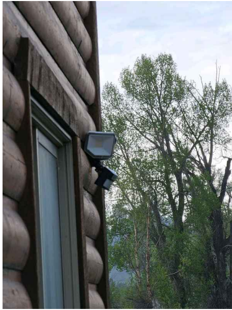
Repaired as of 5/29
