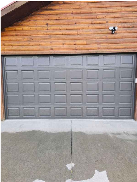
Repaired as of 5/29
