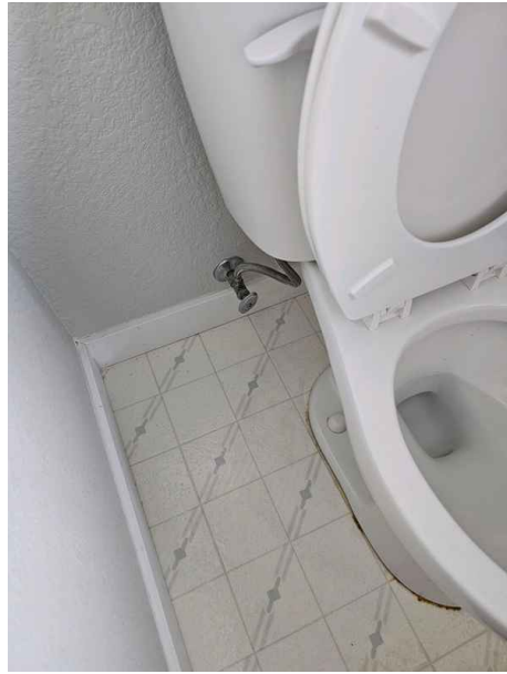
Repaired as of 5/29
