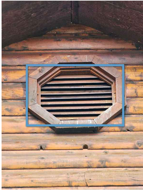
Repaired as of 5/29
