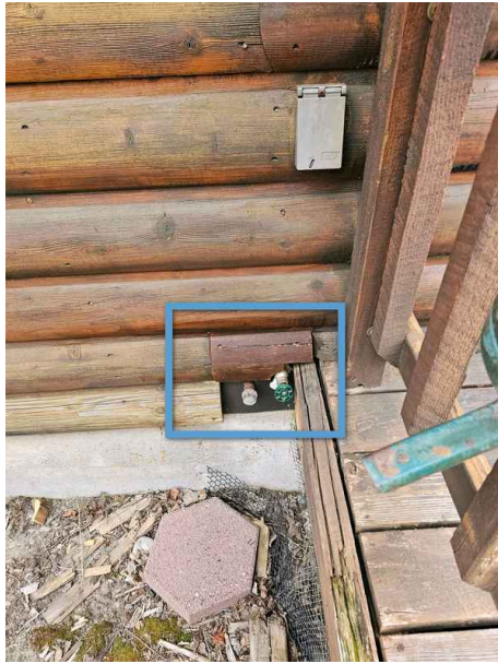
Repaired as of 5/29
