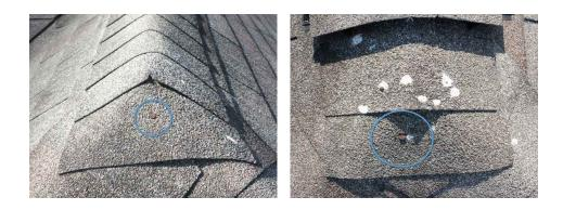
2.3.4 - I. Structural Systems: C. Roof Covering Materials SHINGLES RIDGE CRACKED
