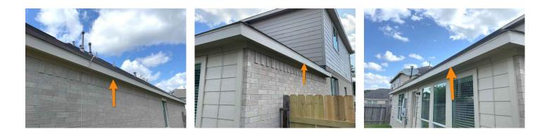
2.3.2 - I. Structural Systems: C. Roof Covering Materials EXPOSED NAILS Maintenance Items/FYI/Minor Defects
