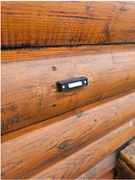
Repaired as of 5/29
