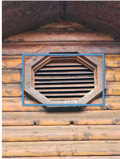
Repaired as of 5/29
