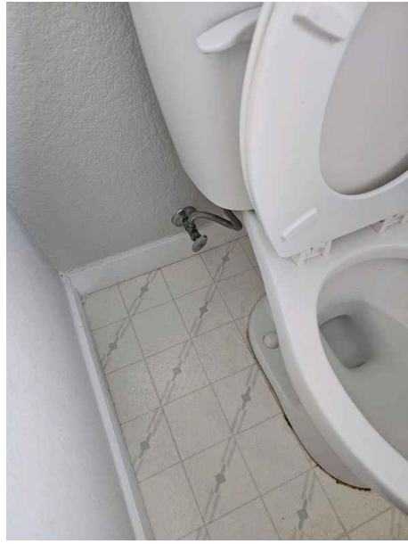
Repaired as of 5/29
