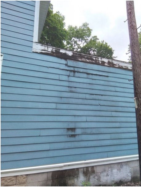
1st Floor right side. No overhang allows roof runoff to run down side of house.
