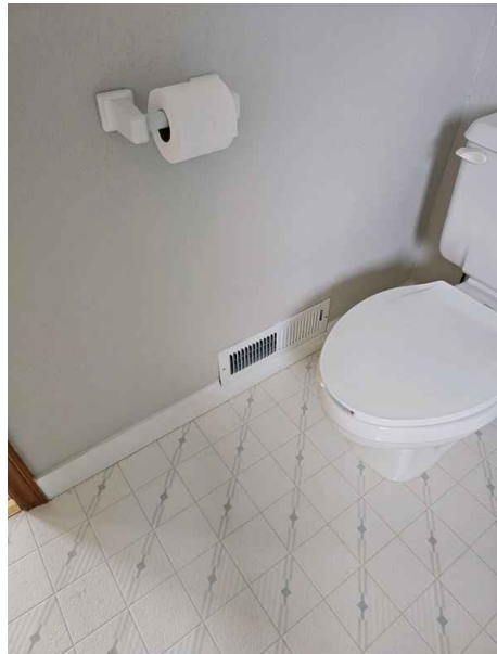
Repaired as of 5/29
