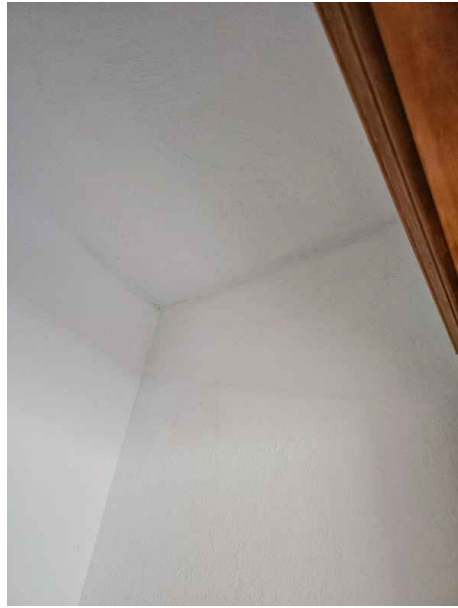
Repaired as of 5/29
