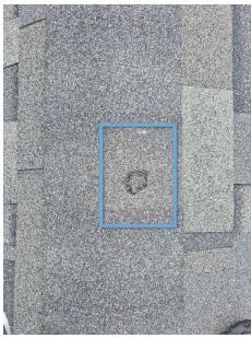
4.2.2 - Roof: Composition Shingle Roof Notes EXPOSED NAILS VISIBLE
