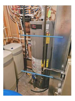
11.1.2 - Water Heater & Plumbing: Water Heating System PIPES-CORROSION
