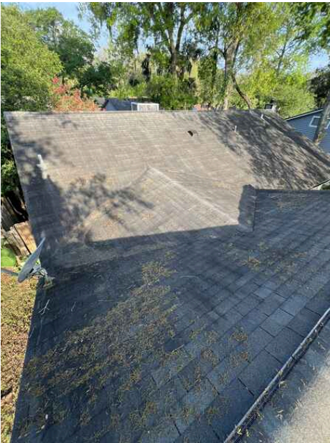
Photos of Each Slope
