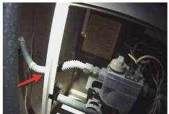
Flex gas pipe is not allowed to be ran through the side of the furnace cabinet. There should be rigid pipe extended from the furnace valve assembly to the outside of the cabinet. A sediment trap is also recommended.
