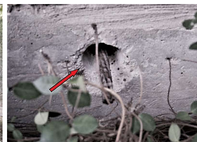
Example Picture of an Exposed Post Tension Cable (Live End)
