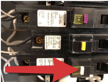
AFCI Breaker for protection from arcing
