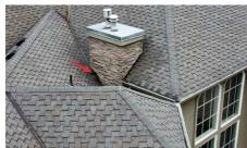
Debris build up along chimney flashing.
