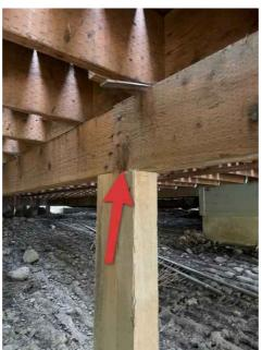
missing post to beam bracket.
