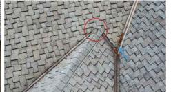
Debris build up in valley flashing. Also damaged ridge cap within red circle.
