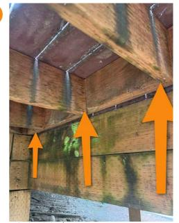
missing joist hangers.
