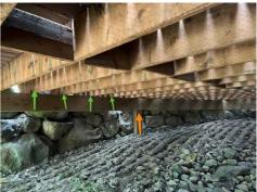
No bracket for post to beam. Also no hurricane straps for floor joists.
