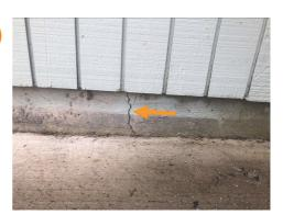
Moderate sized cracks were observed on the Exterior foundation. This suggests unstable or settling soils. Recommend a soil or structural engineer should be consulted for corrective repairs. This may include sealing the pieces back together with a concrete or similar patch. Sealing is to deny possible moisture entry. a structural engineer evaluate and provide a report on course of action and remedy.
