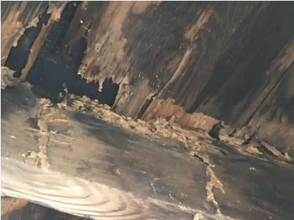
Termite Damage
