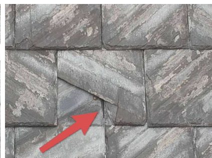
Broken, exposed gap between tiles
